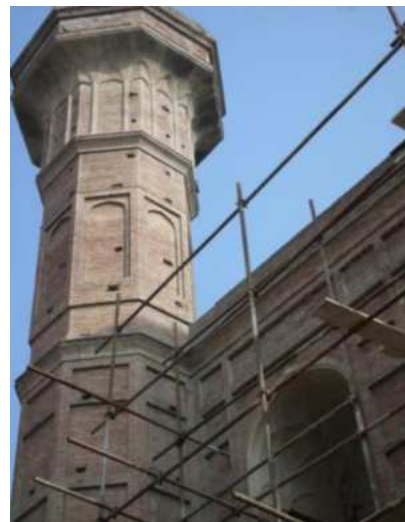
Fig.14 Scaffolding on Minaret of Chauburji
