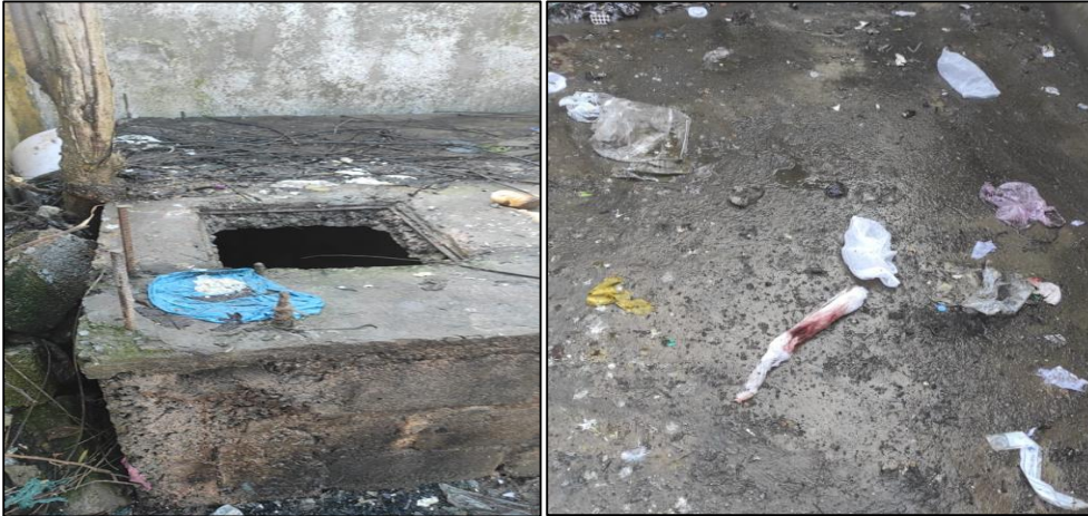
Figure 04 Operation theatre waste in an underground tank
