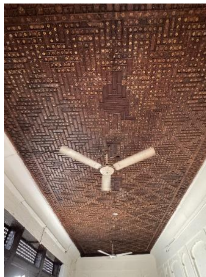
Figure-7 wooden ceiling with mirror in the center (Source: Author)
