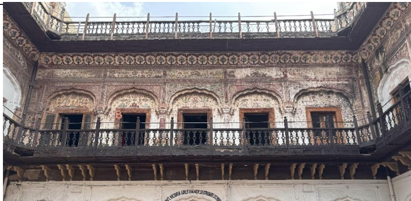
Figure-10. Interior courtyard details of Nau Nehal Singh's Haveli, Lahore. (Source-Author)
