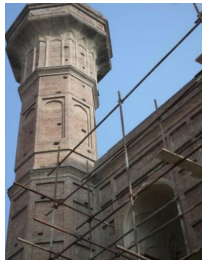
Fig.14 Scaffolding on Minaret of Chauburji
