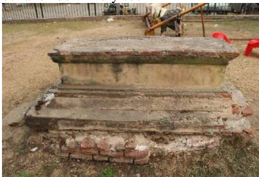
Plate.37 Damaged grave located inside the garden of Mahābat Khān.
