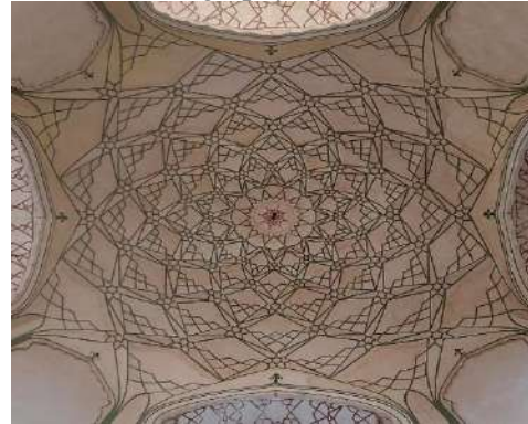
Plate.13 Renovation work at the interior of the tomb of Nādrah Baigam, Dharampura, Lahore Source: Photography by the author.
